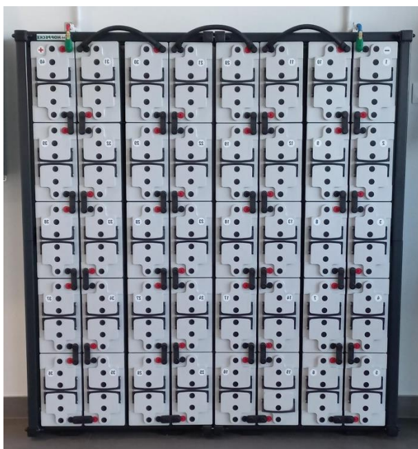
6-3 - Example of horizontal battery arrangement
