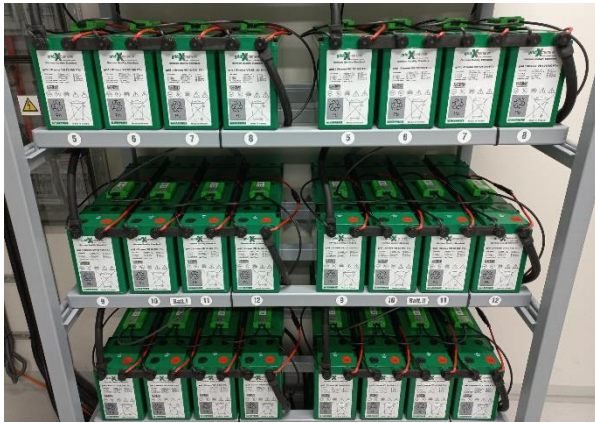
Figure 6.6.5-1 - Use of series and step connectors
