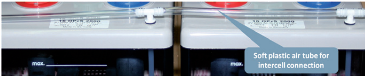
Figure 10: Connection between air tubes - I
