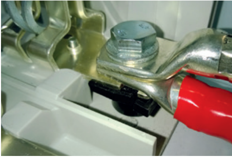
Figure 12: Parallel connection of the sun.fusebox NH2
