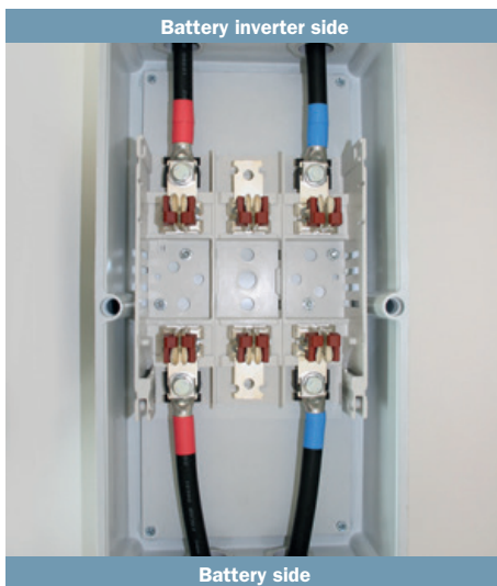
Figure 11: Connecting the sun.fusebox NH2
