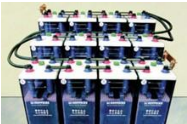
Figure 6.6.5-1 - Use of series and step connectors
