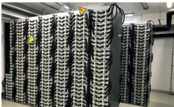
6-4 Example of horizontal battery assembly with grid | power VR M on a rack
